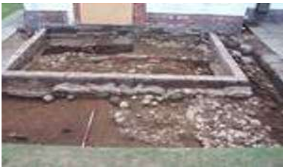
The conservatory trench
