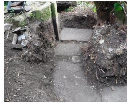
Doorway 2nd from west
