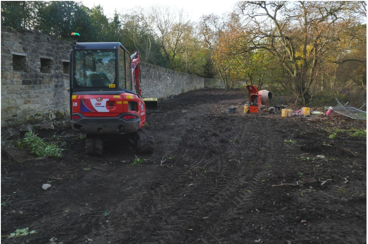
WALLED GARDEN, SOUTH WALL, CONSOLIDATION IN PROGRESS
